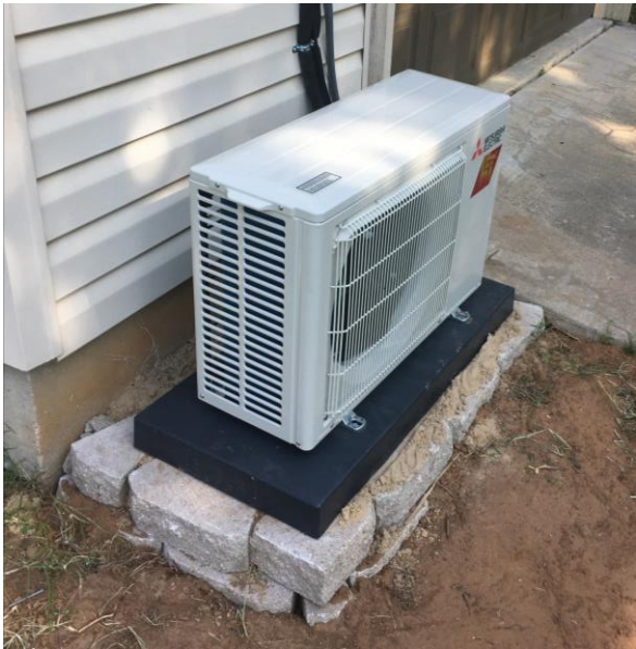
Twin Minisplit HVAC Units Were Installed, Centered On the North and South Walls
