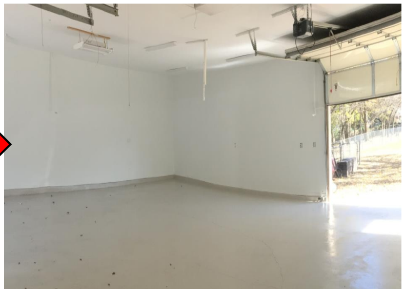
The Shop Walls Were Painted and the Floors Painted With Epoxy
